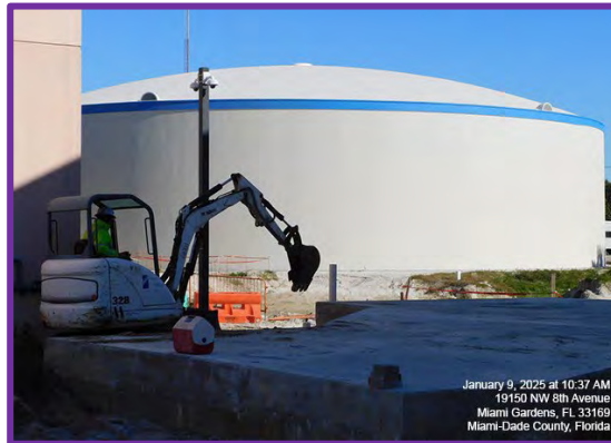
Norwood Water Treatment Plant – 5-Million-Gallon Water Storage Tank
