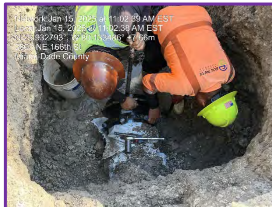
Eastern Shores Watermain System Rehabilitation – Phase 2
