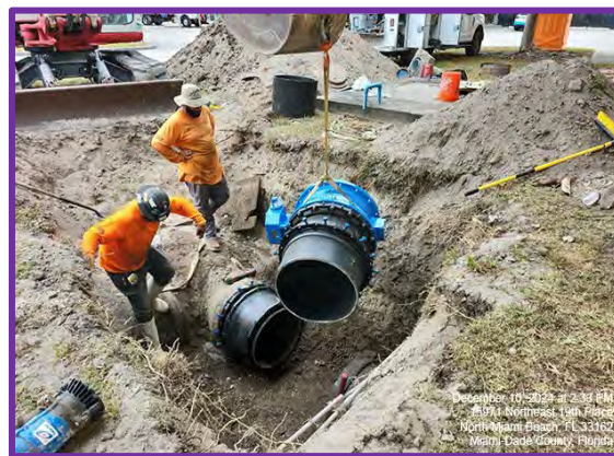
NMB Water Operations Center Rehabilitation
