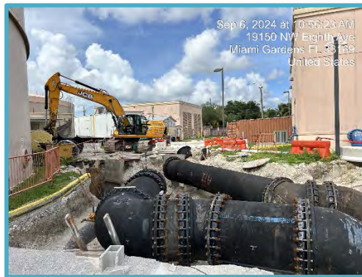
Norwood Water Treatment Plant – 5-Million-Gallon Water Storage Tank
