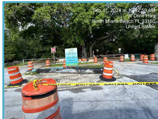
Oleta River Crossing Watermain Replacement
