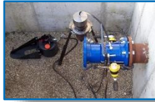
Medium and high pressure system: Resin injection connection
