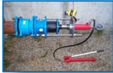
Low pressure system: Mechanical clamping connection
