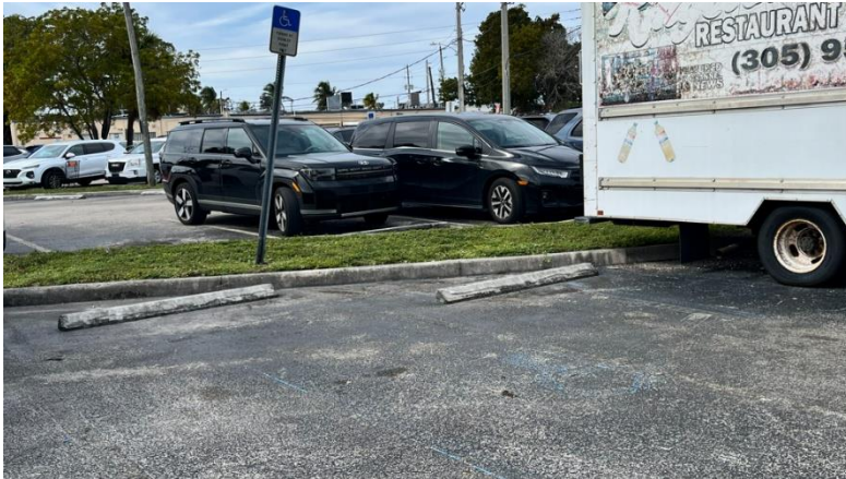
FIGURE 4: IMAGE OF AN ADA PARKING SPACE WITH SEVERELY FADED AND/OR MISSING/INCORRECT MARKINGS
