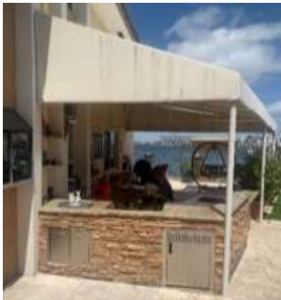
Photo of the awning at 2811 NE 164 th St. Unit 1.
