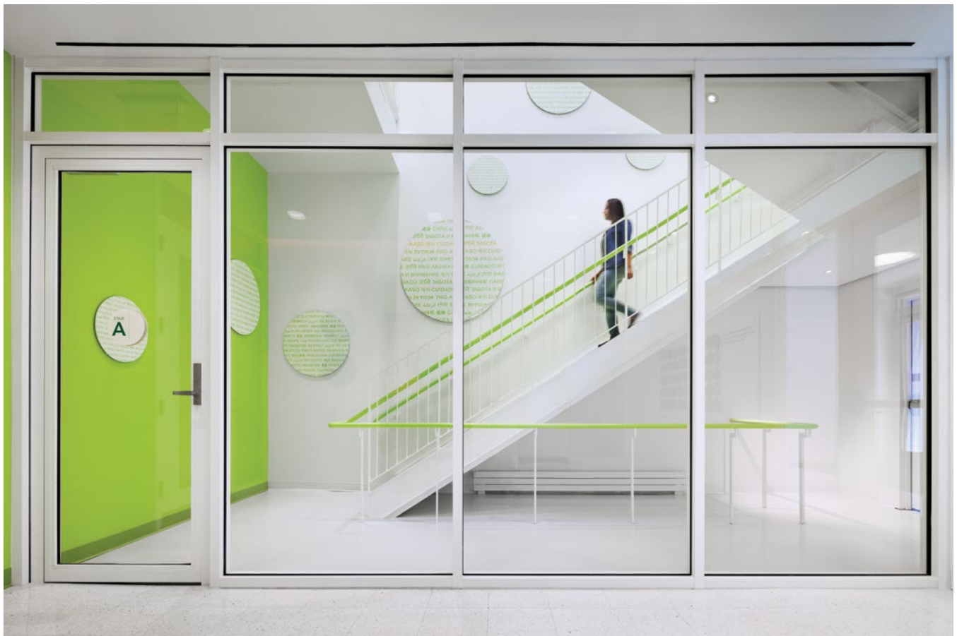
Fire-rated glass, natural light, and colorful graphics transform ordinary fire stairs into light-filled communicating stairs at Planned Parenthood of New York City in Queens, New York.
