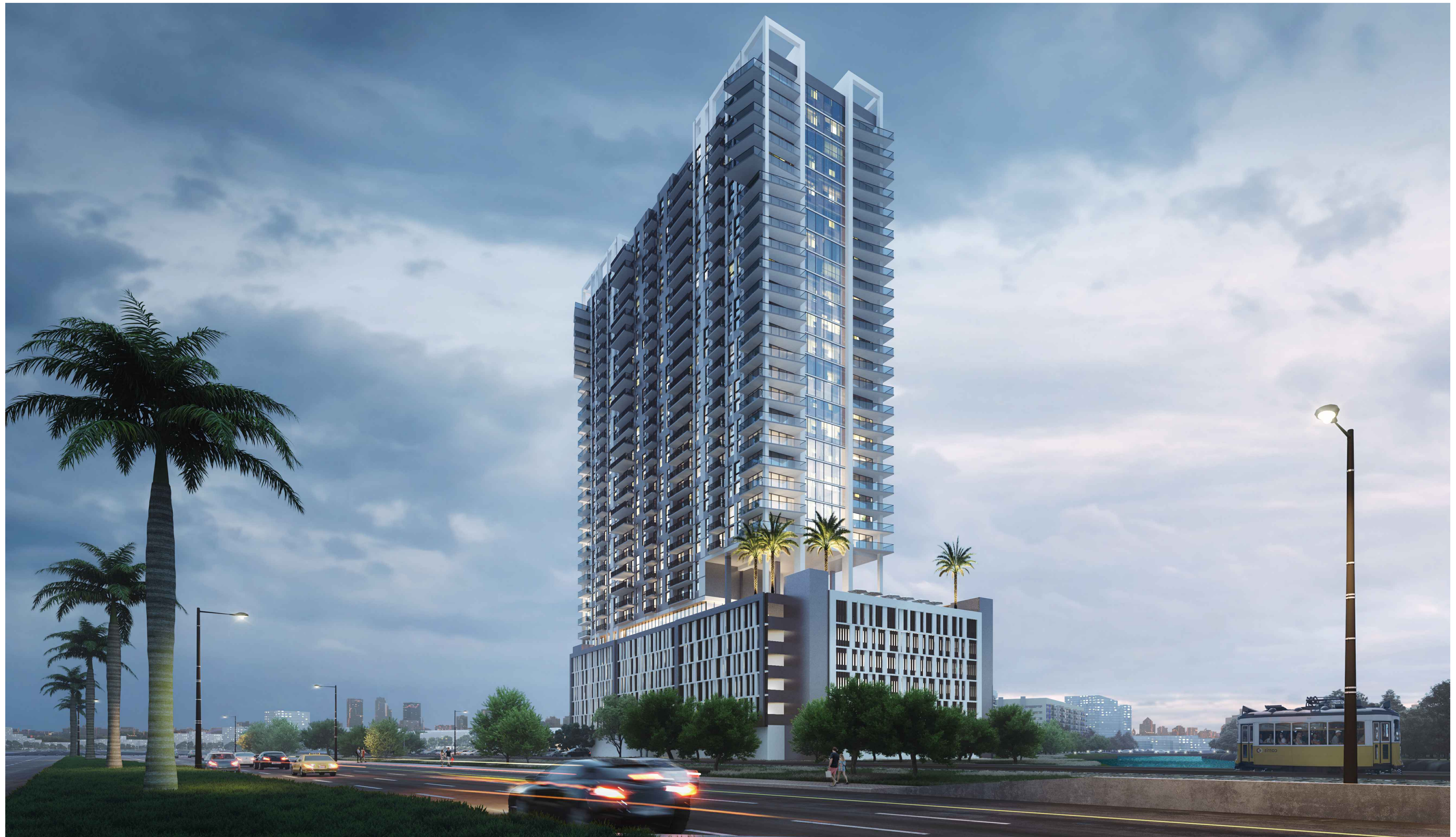
VIEW LOOKING SOUTH
