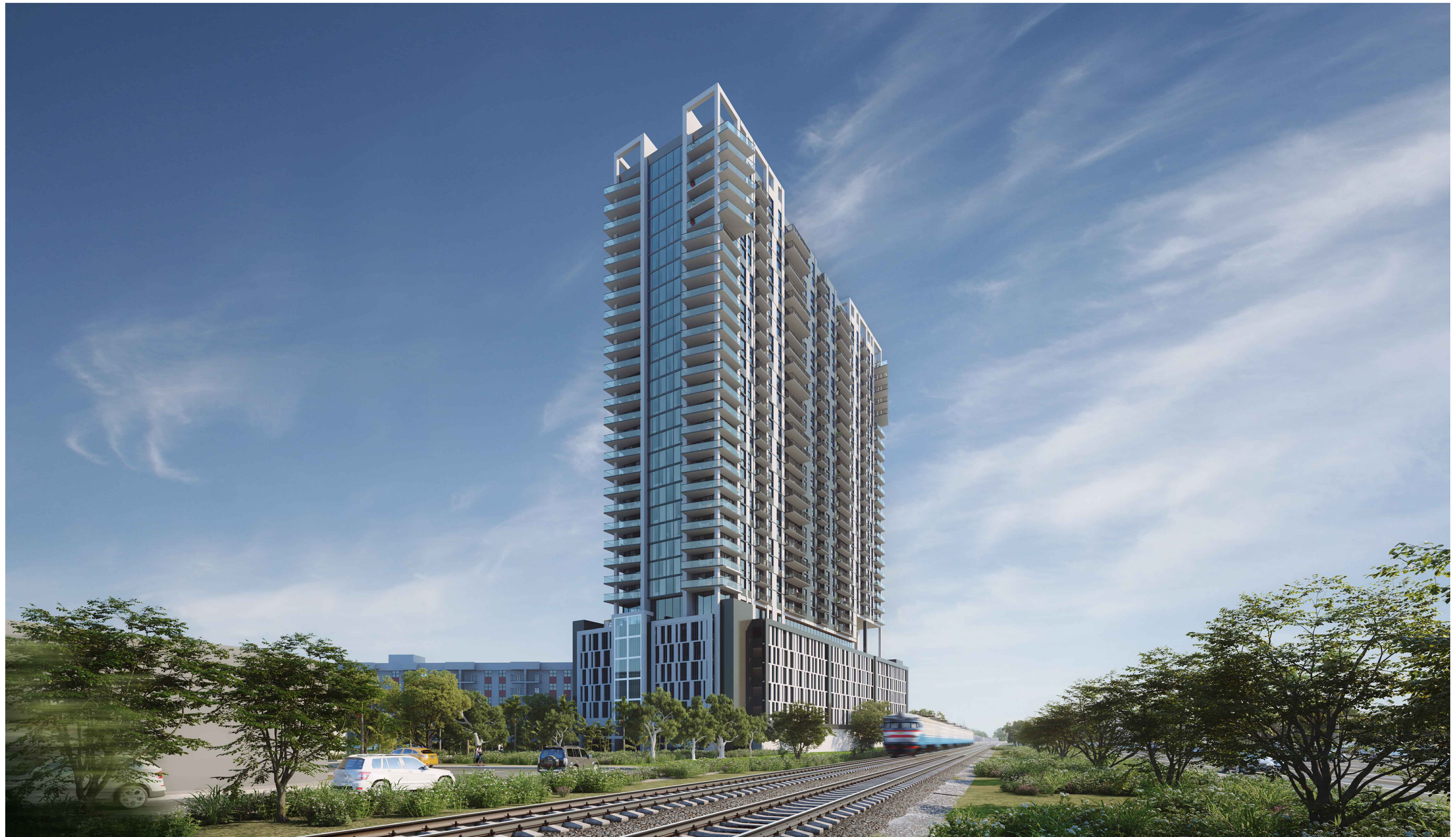
VIEW LOOKING NORTH
