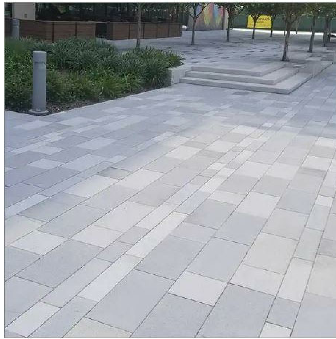
4. PAVERS/HARDSCAPE: WAUSAU TILE - H SERIES PAVERS RANGE IN THICKNESS FROM 1 5/8" - 4" DEPENDING ON THE SIZE. EACH WAUSAU TILE PAVESERIES IS ALSO AVAILABLE IN AVARIETY OF STANDARD AND CUSTOM PLANK-STYLE PAVESERIES.
